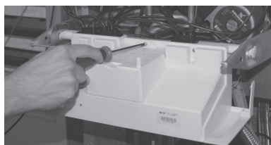
Screw the terminal box cover on tight
