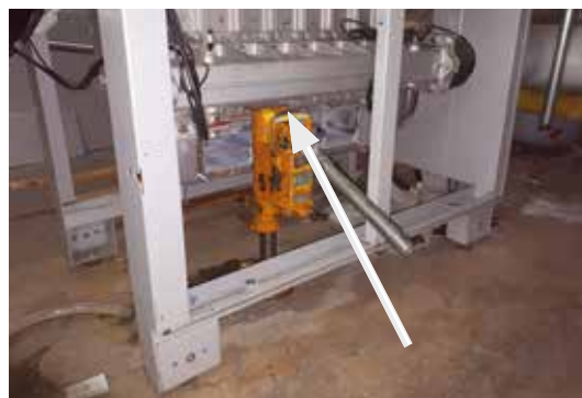
Jack beneath return pipe
