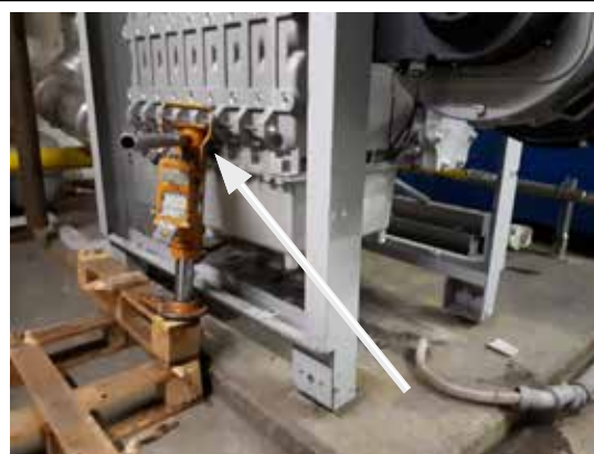
Jack beneath connecting rod
