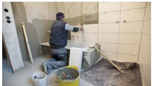
Tiling and sanitary installations
