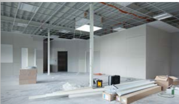
Drywalling and electrical installation
