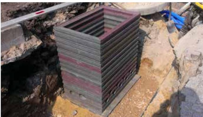
The modular substructure segments reduce installation costs.
