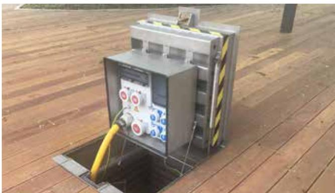
Easy to open with the support of pneumatic springs.
