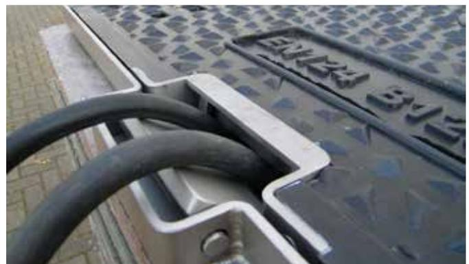
The cables are led to the outside when the cover is closed.
