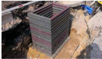
The modular substructure segments reduce installation costs.
