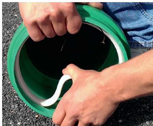
Insertion of the welding ring.
