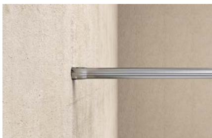
Hohlbohren in Betonwand
