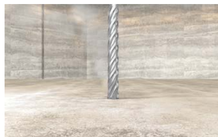
Bohren in Bodenplatte
