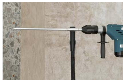
Bohren in Beton
