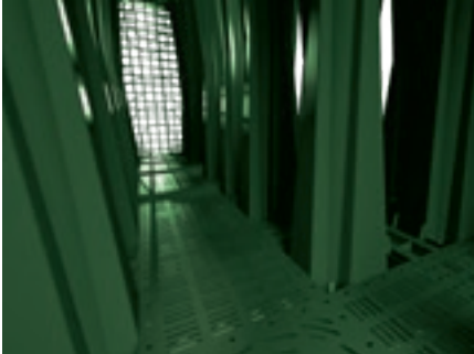
Cross-shaped inspection/maintenance tunnel
