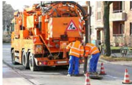
The material like sludge and sand as well as the flushing water taken out of the tank may contain hydrocarbons and heavy metals. These have to be disposed of according to the local regulations.
