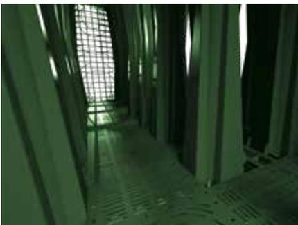
Cross-shaped inspections-/maintenance tunnel
