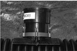
Insert the Aqua-/RobuDock Connecting Set into the hole in such a way that the supporting ring (saddle) rests evenly on the outer diameter of the pipe.
