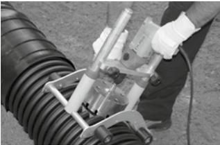
The opening of the main pipe should be made with a suitable hole saw ( $\varnothing 178,5 \pm 0,5$  mm) including guide drill. We recommend the hole saw that is part of our range of products.
