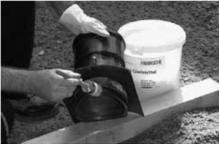
Please ensure that the Aqua-/RobuDock Connecting Set is free of dirt. Apply enough lubricant (FRÄNKISCHE) to the outer surface of the pressure connection (see picture to the left).
