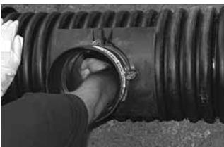
Insert your hand through the opening of the Aqua-/RobuDocks and check the location of the sealing ring.
