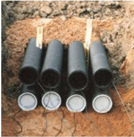
Kabuflex S – spacers indicating the direction make installations fast and safe
